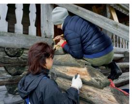
experts conducted a one-of-a-kind operation to lift the church, using a dedicated technology that involved partial replacement of some lower rows of logs without removing them all. In 2008, a team of local carpenters performed a series of restoration works on the bell tower and the roofing.
