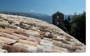
with historic tiles. The project relied on traditional regional building methods – using cypress trees as timber for the ceiling beams from an area nearby, applying traditionally manufactured lime-based mortar, and reusing original tiles when possible, supplementing them when necessary with tiles salvaged from ruins in the region.
