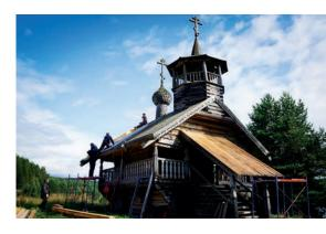
the *okhlupen* – the upper, concluding beam of the roof, which is a typical element of the traditional wooden architecture in the Russian North.
